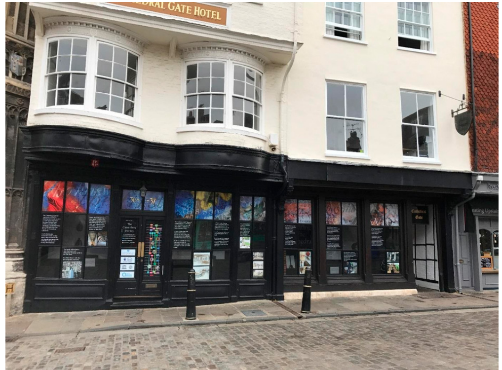
Display in the window of the future Visitor Centre
